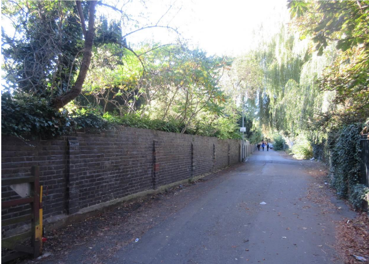
Figure 3: Wall in Quakers Lane
